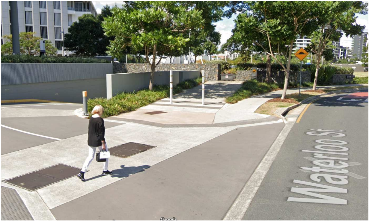
Figure 7 - Google Streetview - Uncompleted bikeway
