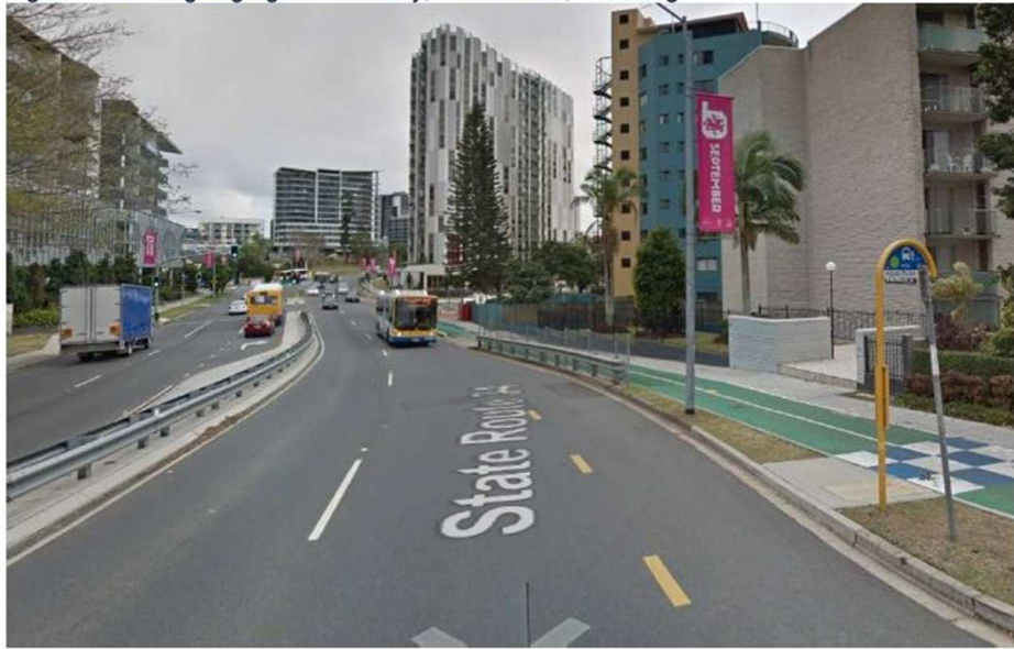
Figure 5: Existing segregated bikeway, Brisbane St, Toowong
