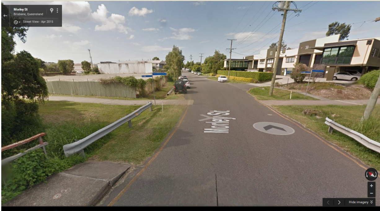
Figure 1: Looking east along Moreley St prior to bridge upgrade
