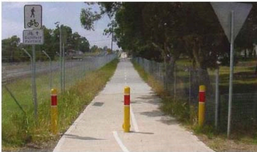
Figure 7.17: Example of a bollard treatment
